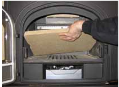
d. Remove the lower baffleplate
